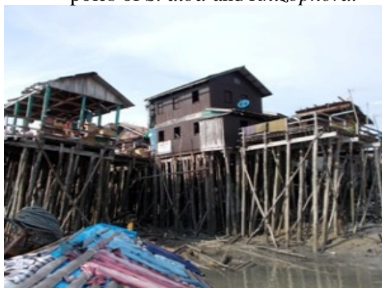
Fig.5. Jetty and house construction by poles of S. alba and Rhizophora .
