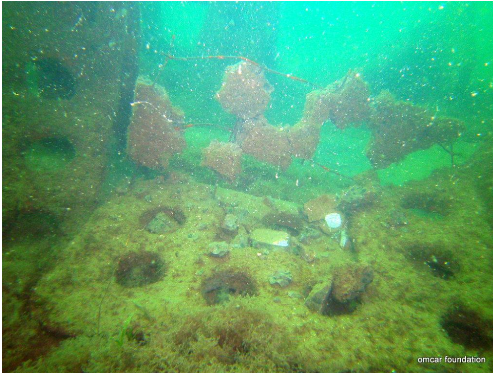
Fig: 49. Artificial reef damaged by dynamite fishing (Jan. 2013)
